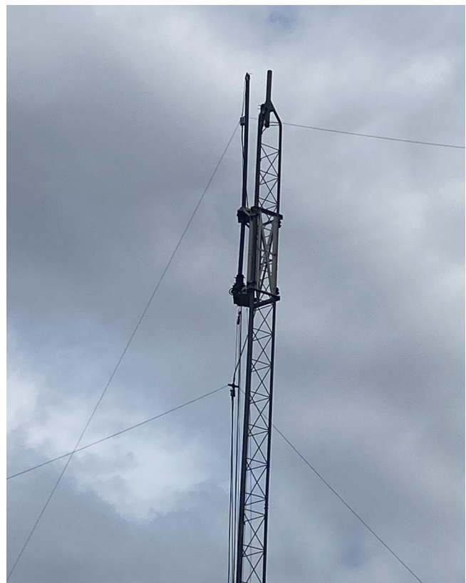
Two dipoles. The top one is at 50 feet and the lower one is at approximately 40 feet.
