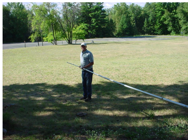
Mast fully extended and ready to be walked up
