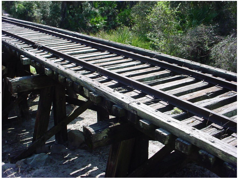
A portion of the original tracks and trestle over a creek
